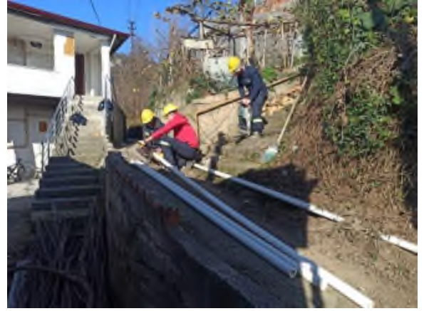
ASMA MAHALLESİ DAĞBACA SOKAK İÇME SUYU HATTI YENİLEME
